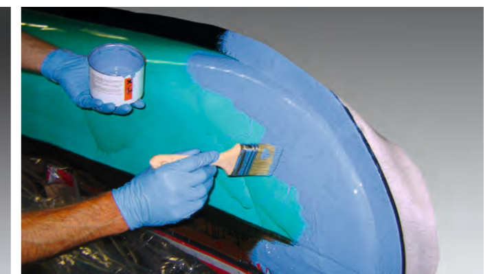
Application of gel coat OH 6-1
