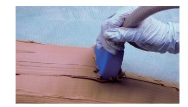
good edge stability, dimensionally stable application of 35 mm layers in one homogeneous surface, good machining
